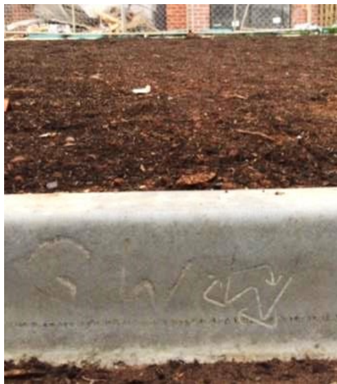
Figure 2: Service Conduit Curb Marker
