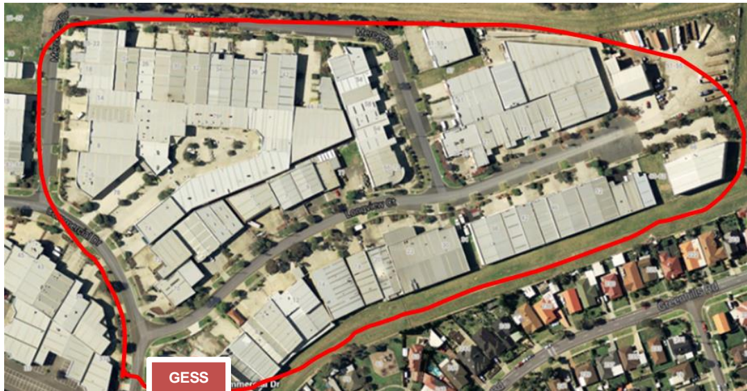
Fig 6: Aerial view of the customers that can be supplied solely by the GESS in 'island mode'
